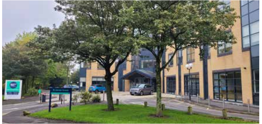
The offices of Granville Credit Control Services are based at St James House, Telford
