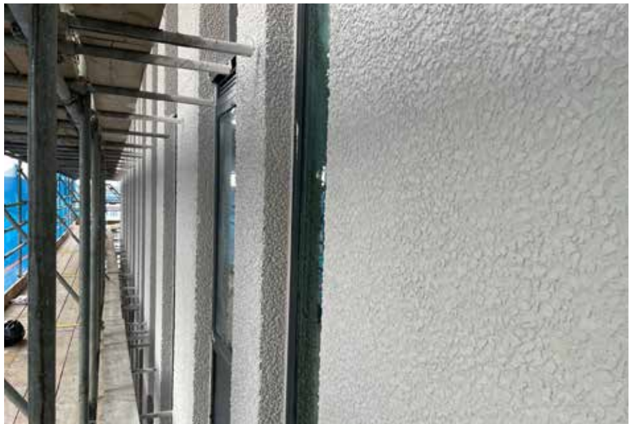
KEIM Soldalit exterior paint applied to the walls of Fairfax House
