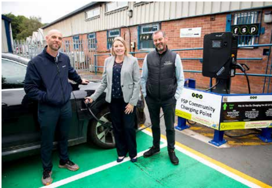
Councillor Carolyn Healy joins FSP's managing director Wayne Carter (left) and chairman, Richard Hilton for the official unveiling of the new EV charging points available for the local community
