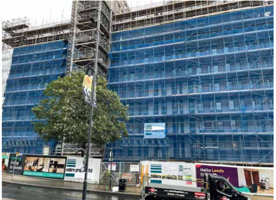
Fairfax House in Leeds has been undergoing a complete renovation
