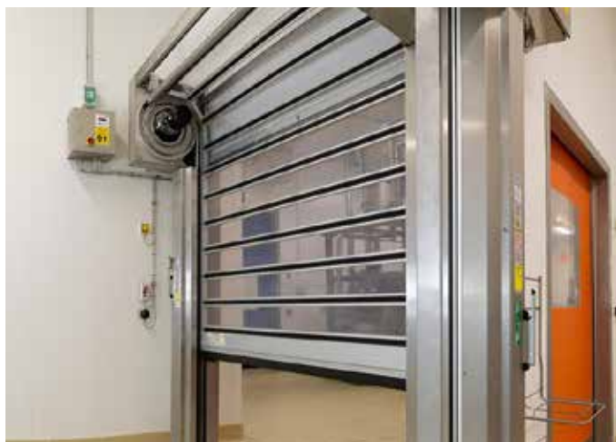
The spiral turbo door has insulation laths and opening speeds up to 3 m/second
